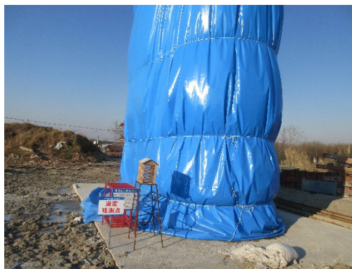
墩柱整体包裹养护
