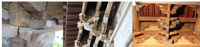
图3 玄贞观大殿半棋、翼型棋、斜棋及铺作里跳翼型棋
