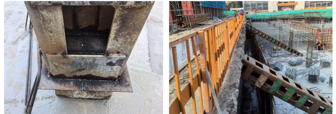
(c) 钢格构立柱及止水钢板焊接
