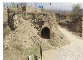
图3南门瓮城修缮前
